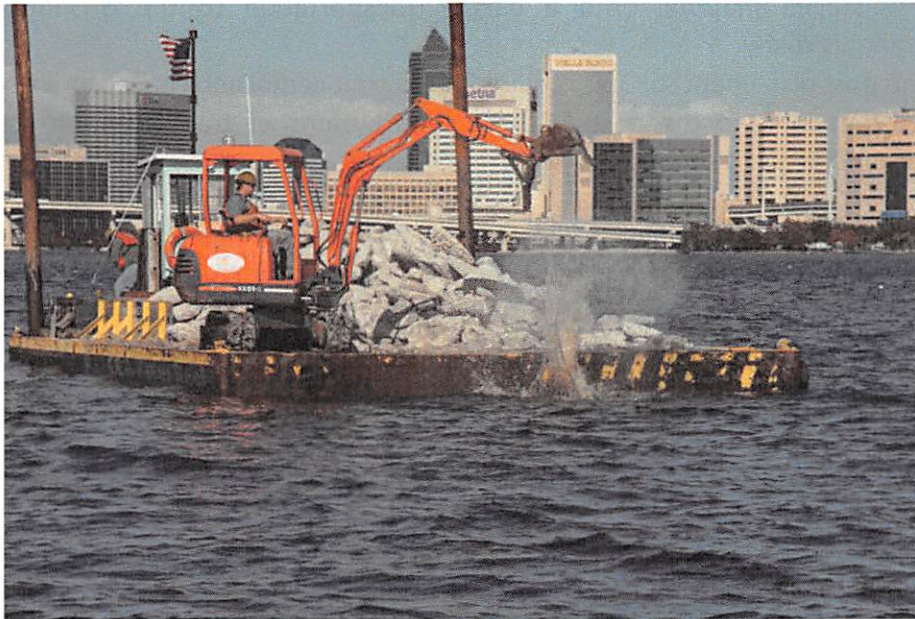
The Community Resident @ http://residentnews.net/2014/12/30/river-project-create-fish-habitat-completed/
